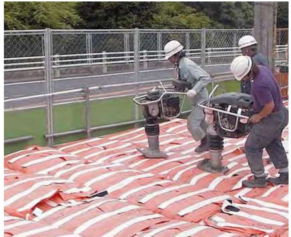
4) Compact D · Box with rammers
