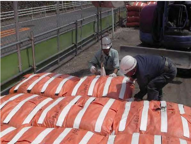
3) Lift the bag with heavy equipment and place neatly
