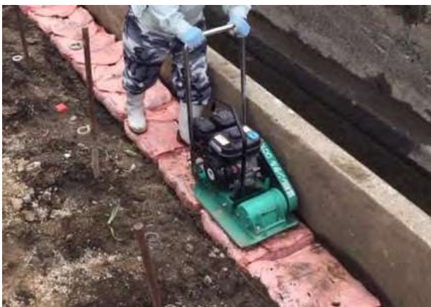
5) Compact with plate compactors until they get tight enough
