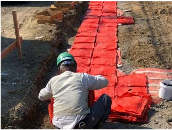
1) Place D - Boxes neatly connecting them with each other using special lock joints
