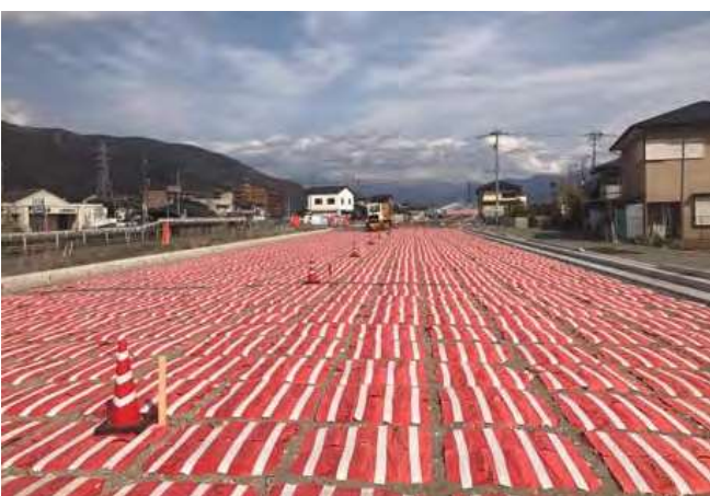
5) An example of works for the ground reinforcement and vibration reduction.
