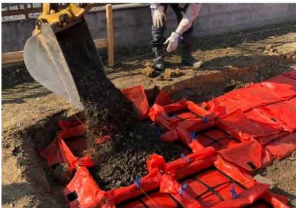
3) Fill fillings, then level its surface.
