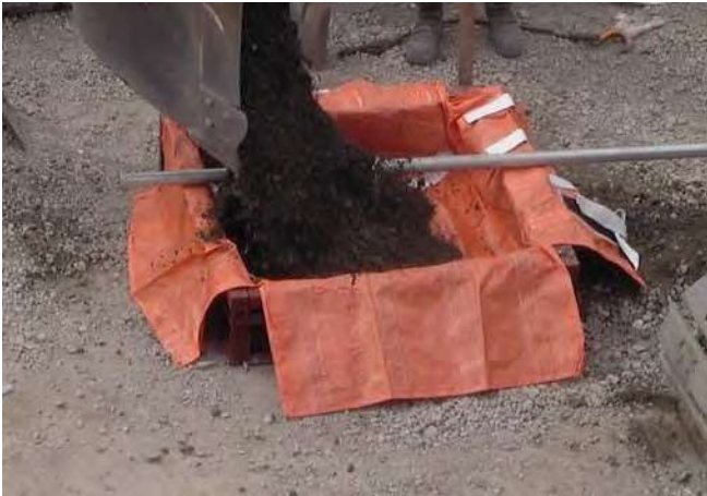
1) Set the D · Box bag in the dedicated frame. Open the bag and pour the filling material.
