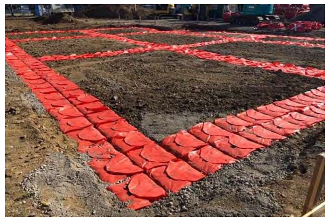
6) Completion example (the picture shows the ground reinforcement for housing constructions)
